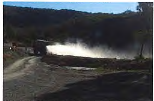
Water cart in operation.
