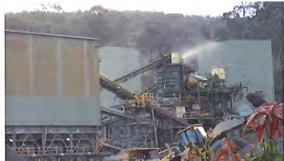
Water sprays and Coolfog™ systems in use that can appear to look like dust, especially in the afternoon sun.
