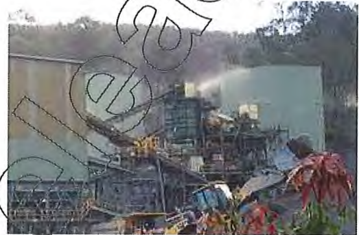
Coolfog in operation.
