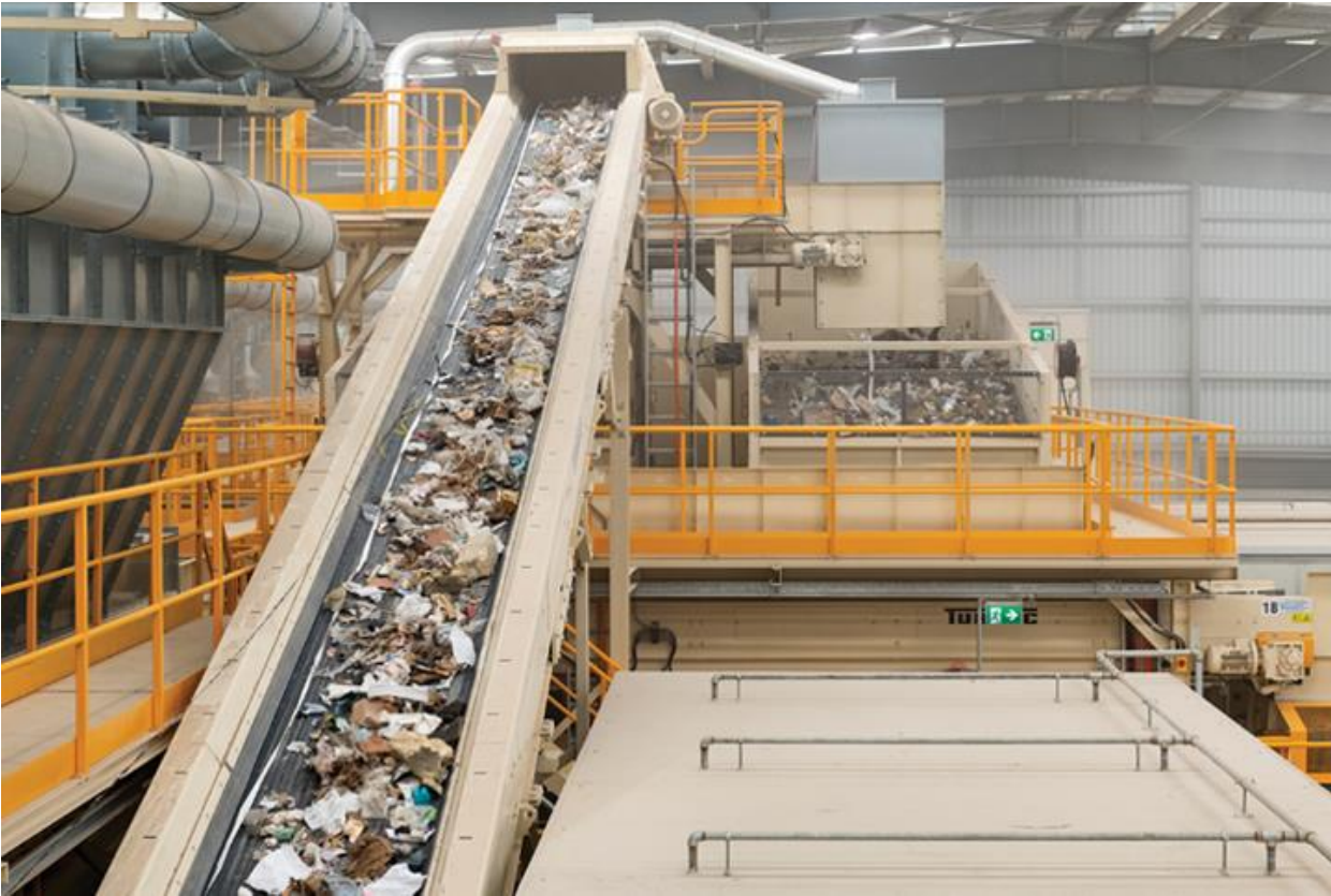
Mechanical sorting of mixed waste feedstocks. Image courtesy of ResourceCo.
