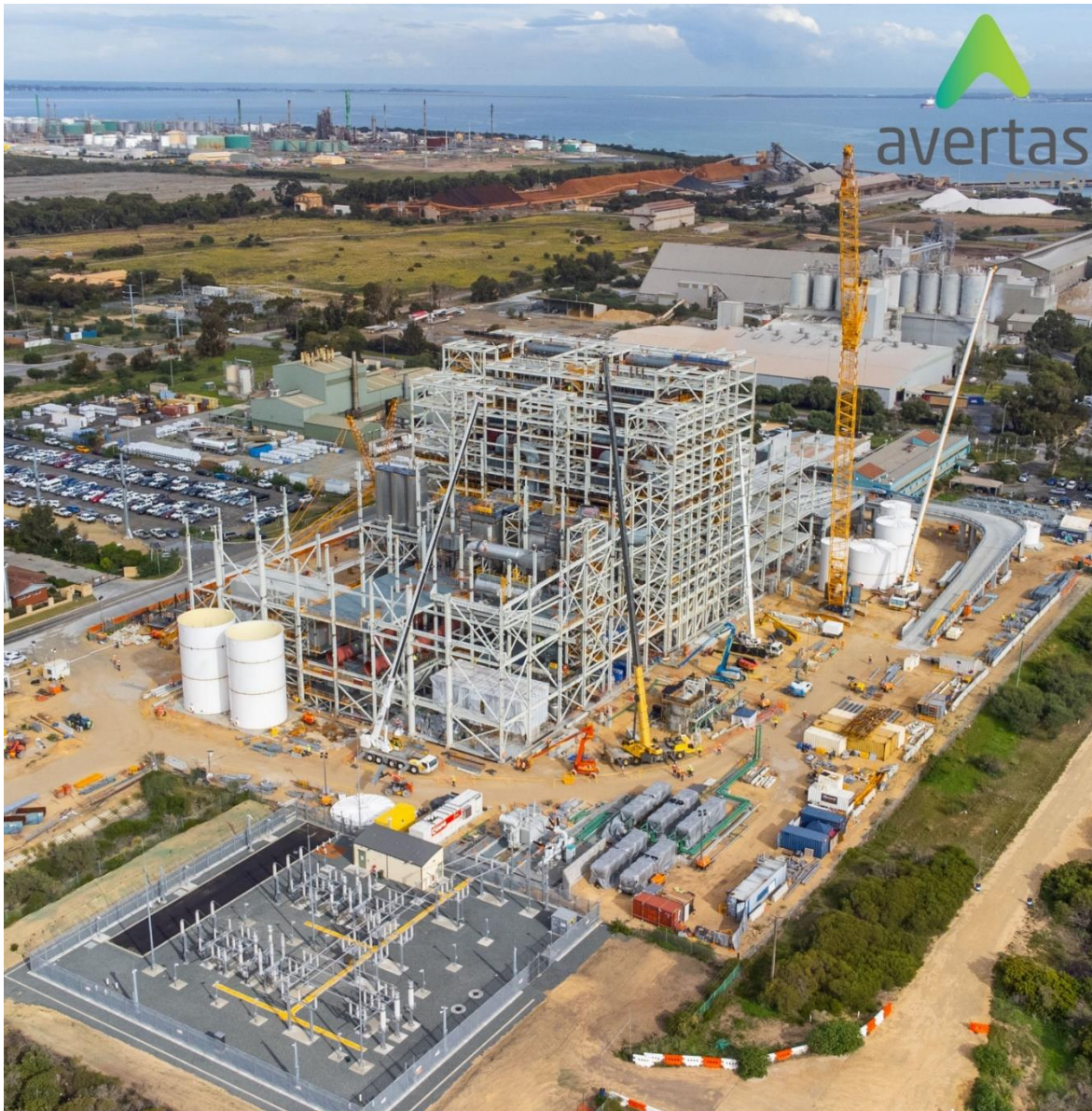
Facility under construction June 11 2021. Image courtesy of Avertas Energy.
