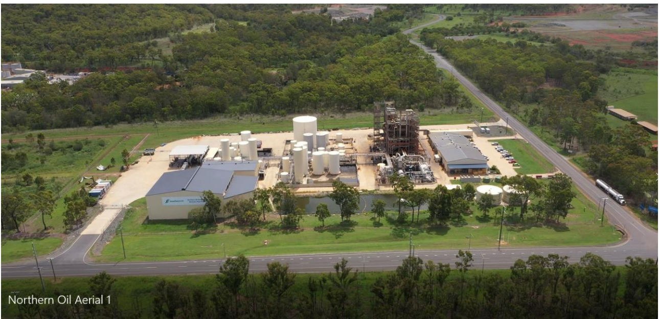
Aerial view of the Northern Oil site. Image courtesy of Northern Oil.
